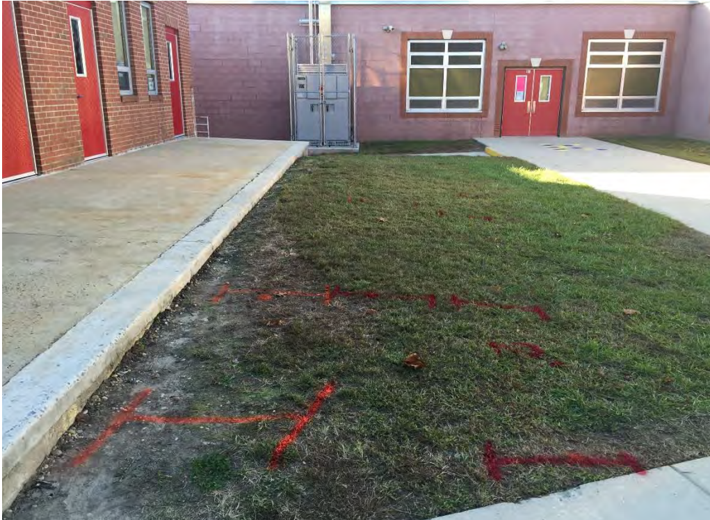
The photo above shows where the above mentioned lines enter the newer portion of the school.
