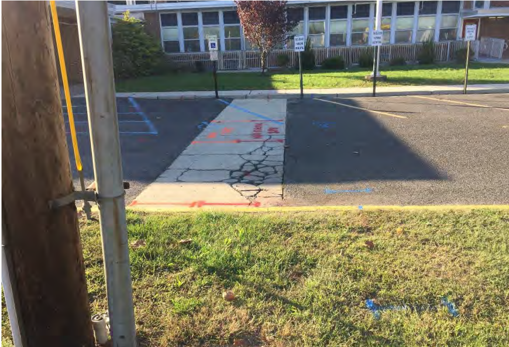
The photo above shows three lines located utilizing the 400MHz antenna and the RD7000. The water line and main electric run parallel to one another across the road.
