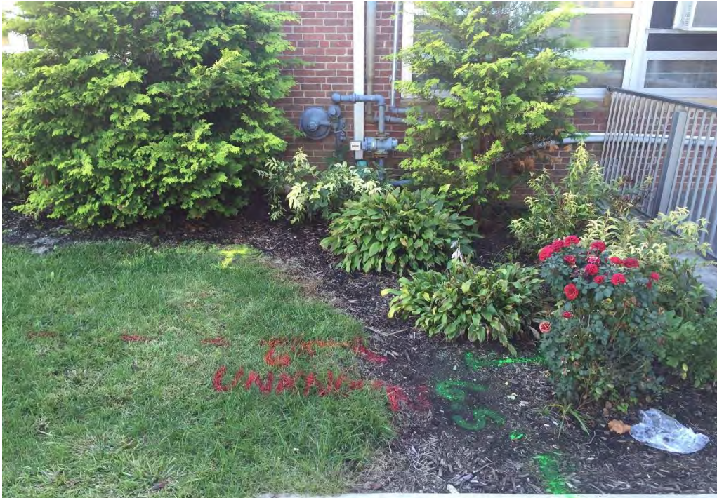
The photo above shows the gas meter on the side of the building. A green paint marking can be seen perpendicular to the building. This green paint indicated the approximate location of the roof drains at 6.5'
