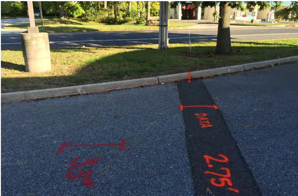
The photo above shows where the main electric and data enter the newer portion of the school building. The electric was located 3.5' subsurface while the data was approximately 2.75'.
