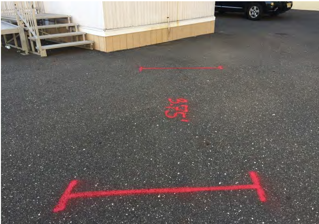
The photo above shows the path the above mentioned conduits take leading into the trailer. These lines were located at approximately 3.75' subsurface.
