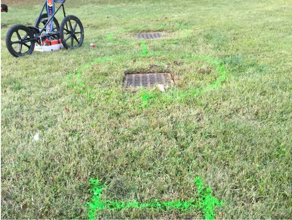
The photo above shows two culverts where the storm drain/roof drains empty into.
