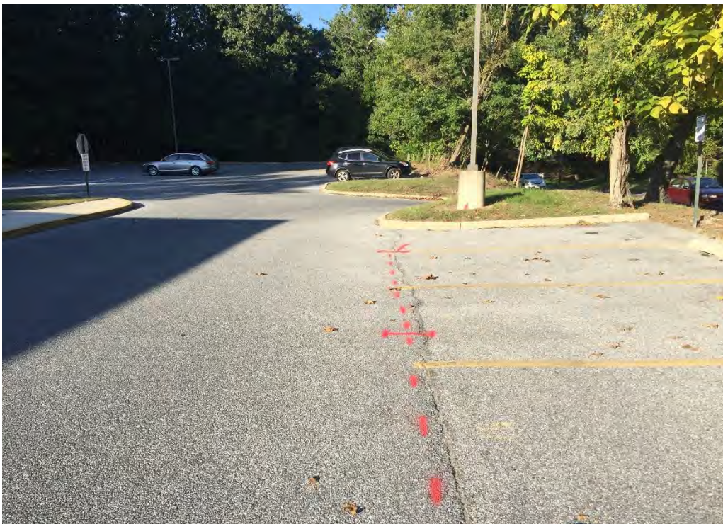
The photo above shows a conduit marked on the surface in red marking paint. This conduit was for the sight lighting located in the parking lot off of Gibbsboro Road.
